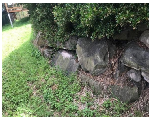
Photograph 5 and Photograph 6: View of degrading retaining wall to the south of the pool.
