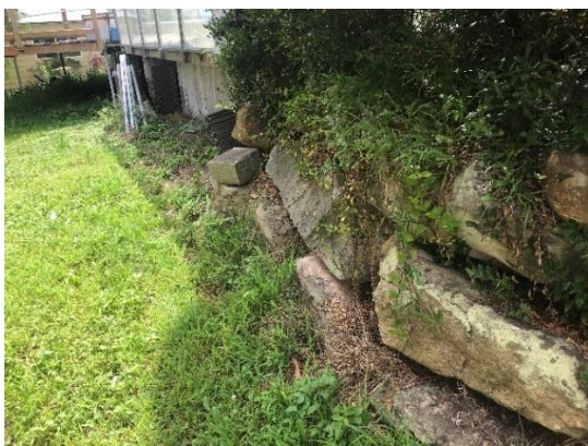
Photograph 5 and Photograph 6: View of degrading retaining wall to the south of the pool.
