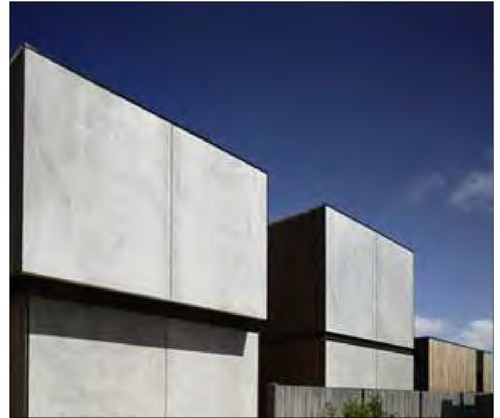
FC - FIBRE CEMENT CLADDING
