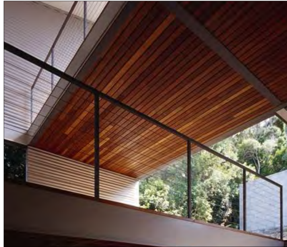
SS - STAINLESS STEEL WIRE BALUSTRADE
