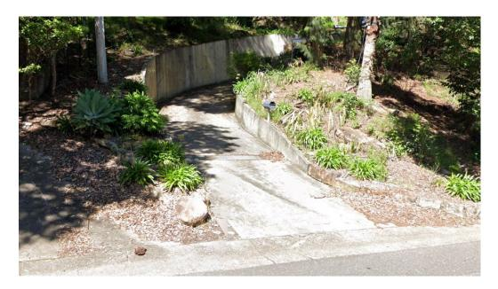
The Internal Driveway shall be contained within the driveway corridor. The minimum width of the driveway corridor (i.e., impervious pavements together with grassed shoulder area) shall be as follows: Single Dwelling: 3.0 metres minimum.
