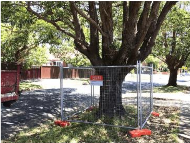
Figure 3 – Example of temporary tree protection
