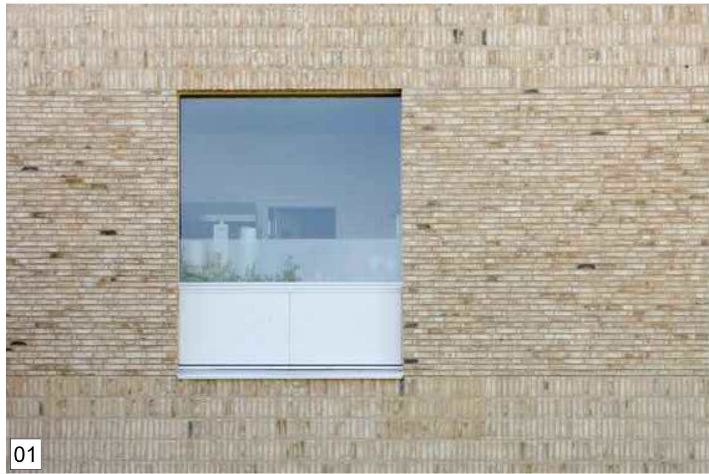
01. BRICK FACADE NUBRIK ARTISAN - AURORA FEATURE SOLDIER COURSING ALONG STREET FRONT FACADE / PERFORATED BRICK PATTERN PROVIDING FILTERED LIGHT TO LEVEL 01 BALCONIES
