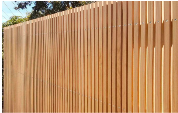
(C) VERTICAL TIMBER SCREEN FENCING
