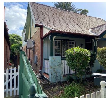
Front Garden – No 12 Subject Site
