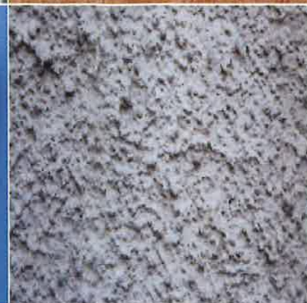
Walling and Slab Edges
