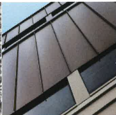
Walling and Eaves Colorbond Jasper Standing Seam
