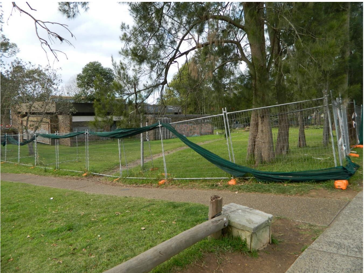
Photograph 2: Subject site, viewed from Lockwood Avenue
