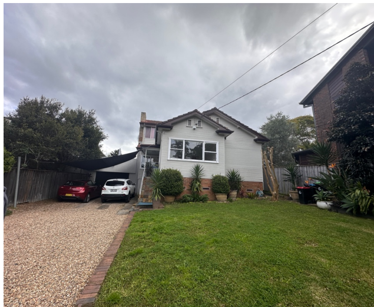
View of Existing Dwelling from Front Yard
