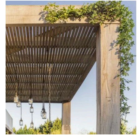
4. Hardwood Timber Pergola and Battens
