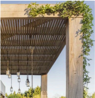
4. Hardwood Timber Pergola and Battens
