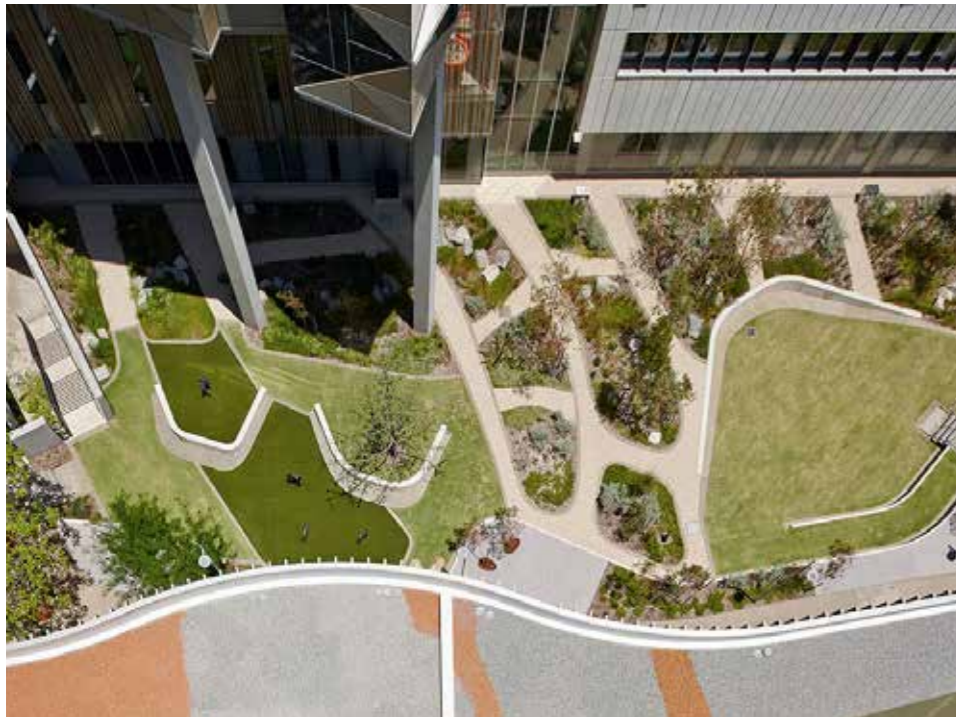
FIONA STANLEY HOSPITAL
