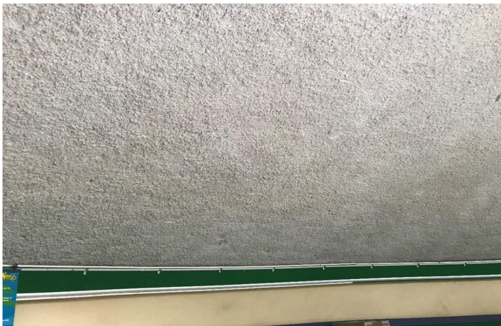
Photograph 1: B00A, R1001 - Storeroom, ceiling , vermiculite, no asbestos detected by analysis.
