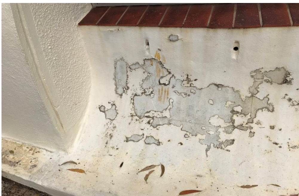
Photograph 2: B00A, exterior, throughout, walls, cream paint , negative for lead.
