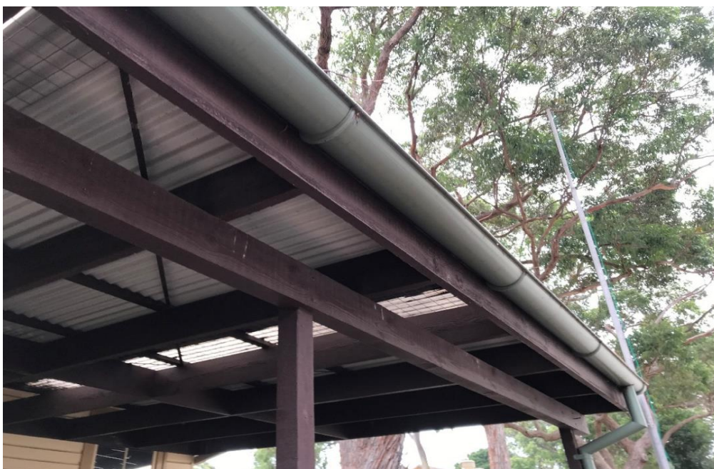
Photograph 5: B00P, exterior, gutters and downpipes, green paint, negative for lead.
