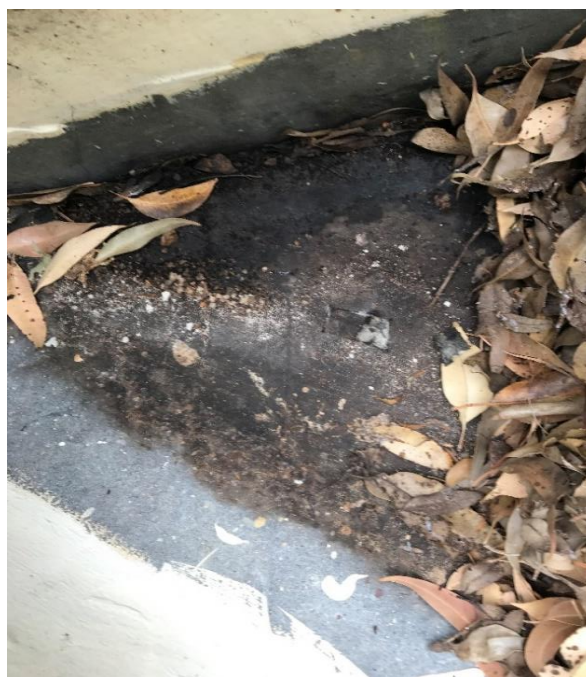
Photograph 4: B00A, exterior, western and north-eastern garden beds, lining to garden bed, bituminous membrane, asbestos detected by analysis.
