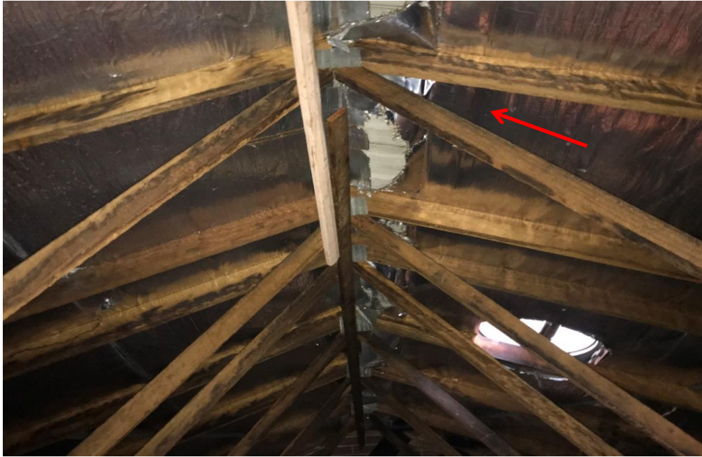
Photograph 5: B00R, interior, ceiling cavity (accessed through R0010), sarking, waterproof membrane , SMF identified visually.
