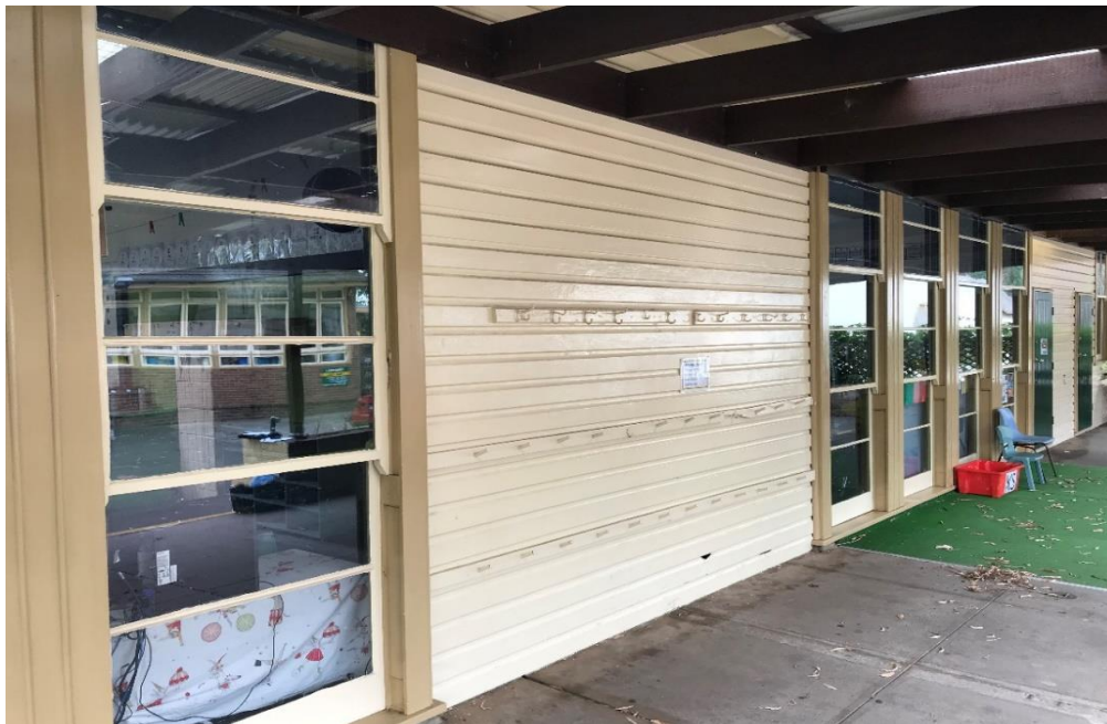
Photograph 2: B00P, exterior, typical wall, cream paint, negative for lead.
