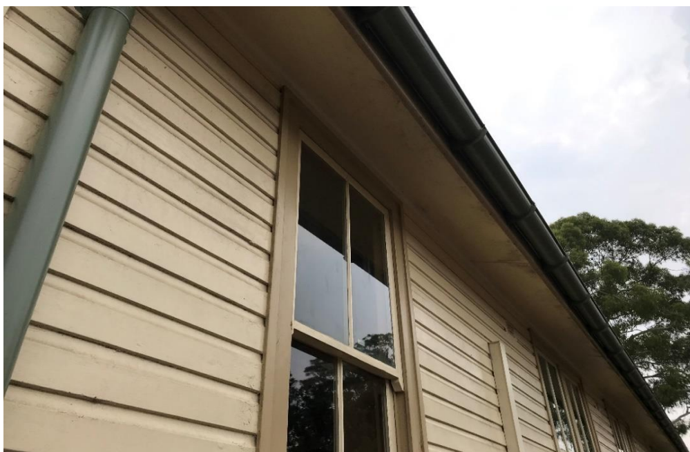
Photograph 4: B00H, exterior , typical gutter and/or downpipe , green paint, assumed negative for lead.
