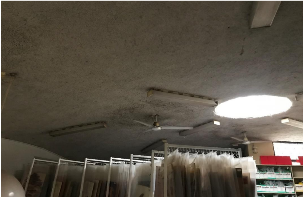
Photograph 3: B00B, R1001 - Special Programs Room, ceilings, vermiculite , no asbestos detected by analysis.
