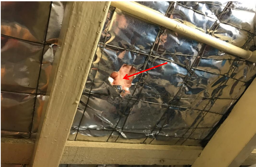
Photograph 4: B00S, R0003 - Ceiling Cavity, underside of ceiling, insulation, SMF identified visually.
