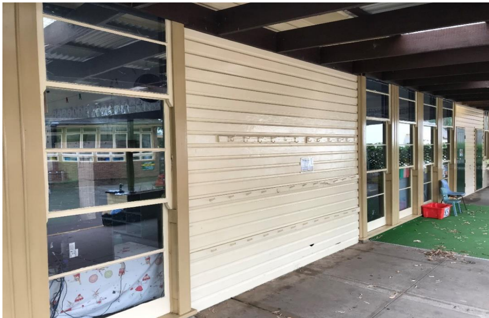
Photograph 2: B00H, exterior , typical wall, cream paint, assumed negative for lead.
