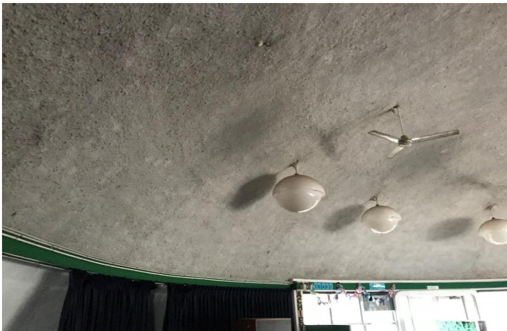
Photograph 2: B00B, R0003 - Reading Area, ceilings, vermiculite , no asbestos detected by analysis.
