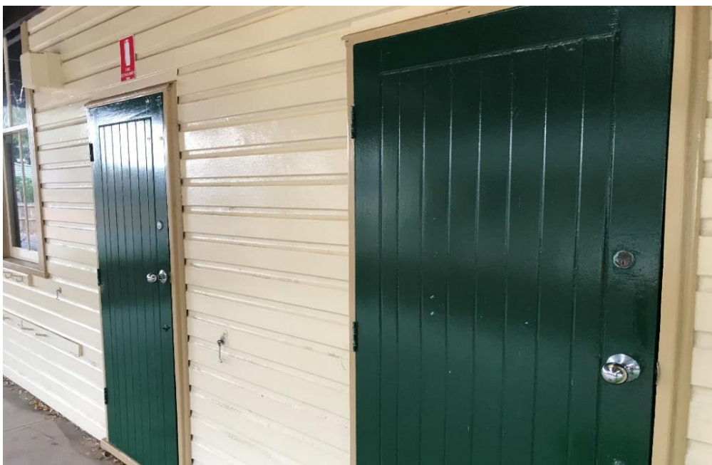
Photograph 3: B00H, exterior , typical door, green paint, assumed negative for lead.
