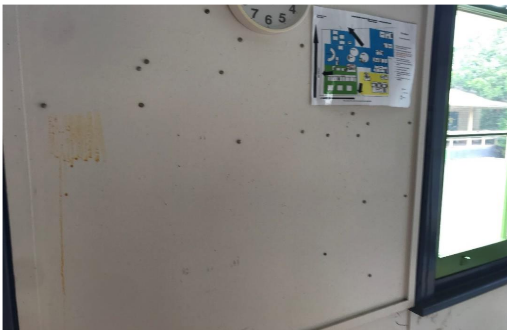
Photograph 5: B00H, interior, typical wall, white paint, negative for lead.
