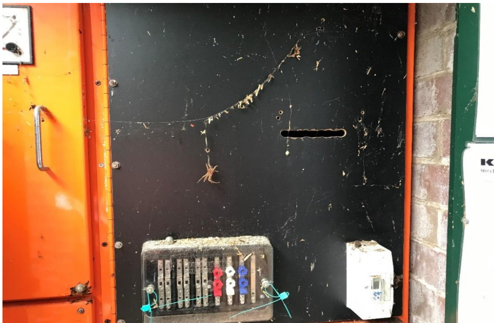
Photograph 2: B00K, R0006 -Distribution Board, electrical distribution board, resinous board, asbestos (assumed).
