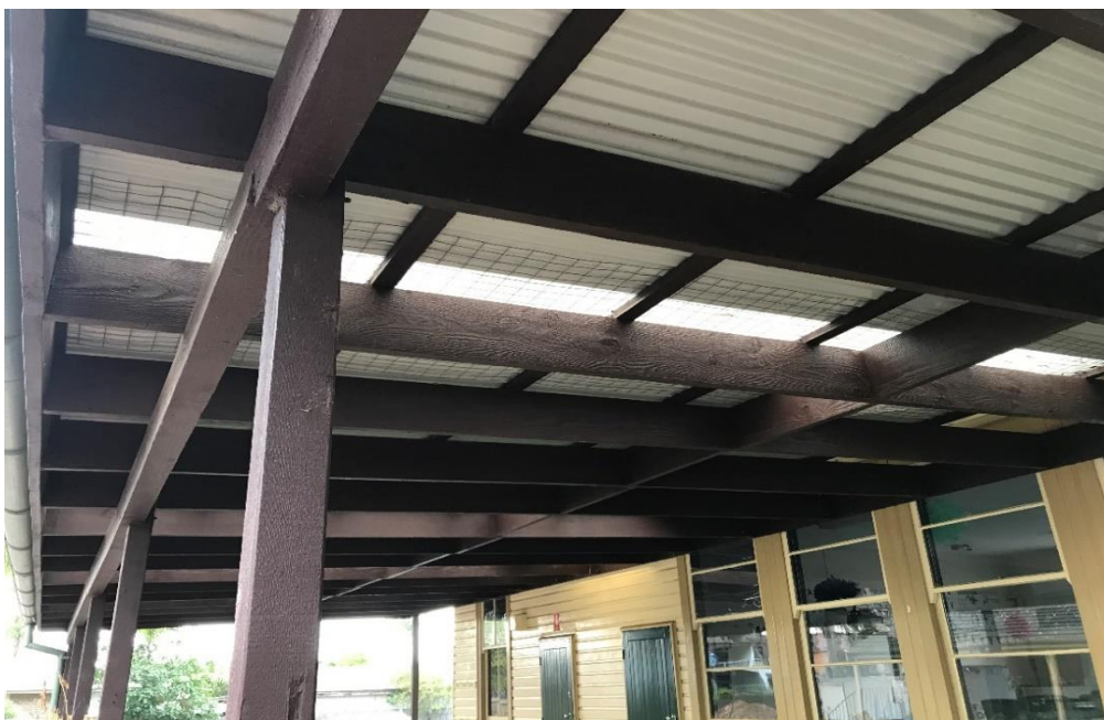
Photograph 3: B00P, exterior, balcony , posts, bearers and joists , typical brown paint, negative for lead.
