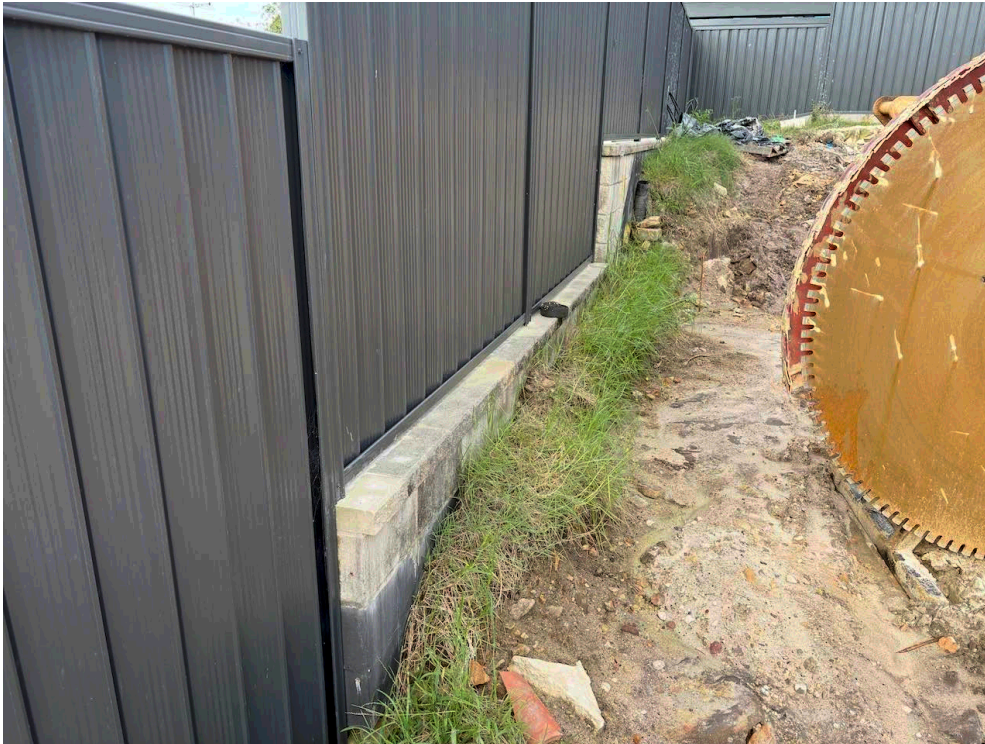
Photo 2: Low concrete block retaining wall and boundary fence, adjacent to the proposed pool excavation.
