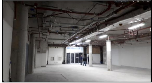
Figure 20. View of internal ground floor facing south east. (Source: mecone, received 23.09.19)
