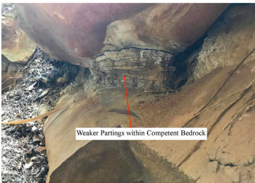
Photograph 12: Weak zones within bedrock
