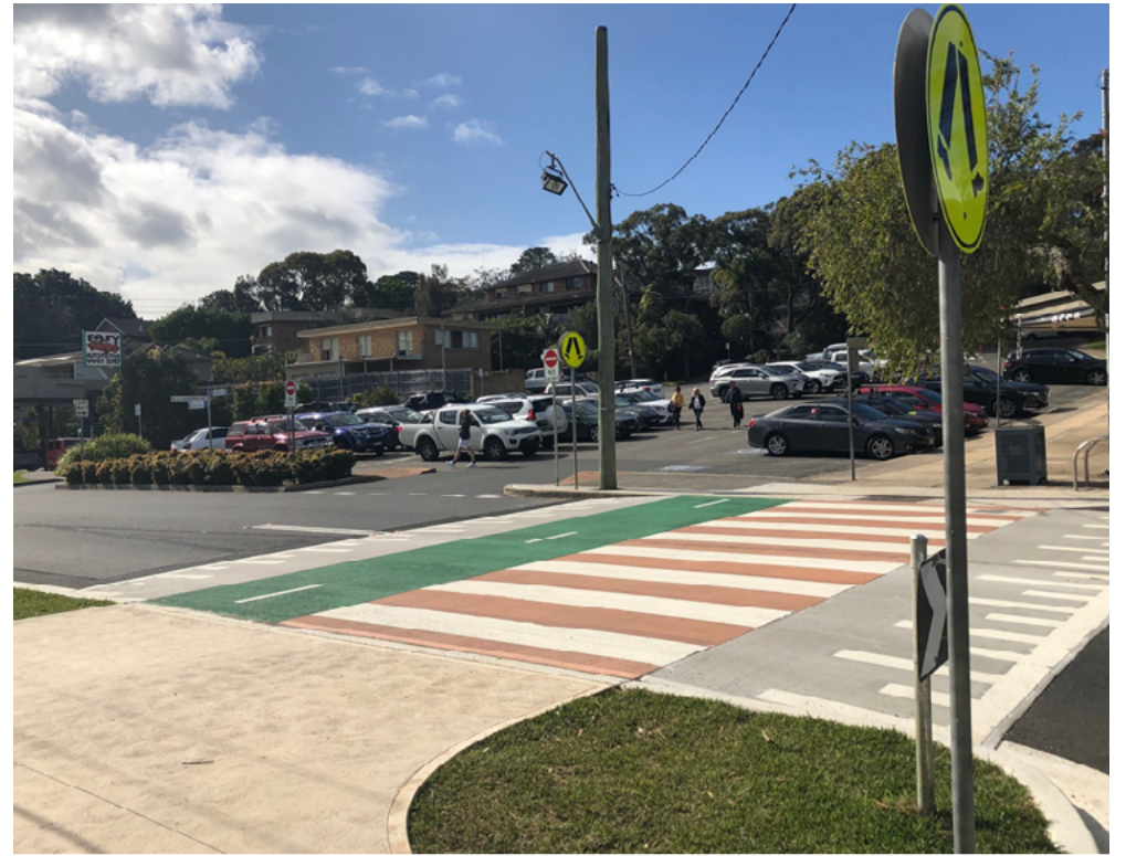
Safer Crossing Treatment, Kalinya St, Newport
