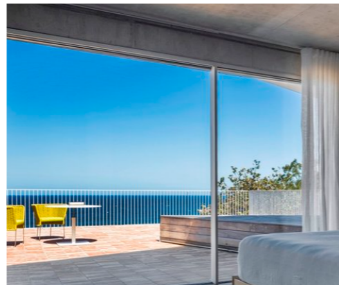
AD & AW - ALUMINIUM FRAME DOOR & WINDOW, TO MATCH DULUX "BASULT" OR SIMILAR
