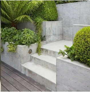
CONCRETE CAST IN STAIRS
