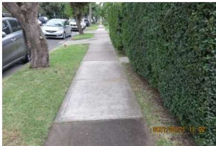
Figure 6: Above confirms previous footpath repair that likely required supporting live roots to be severed. Below illustrates poor pruning practices undertaken over the long term.
