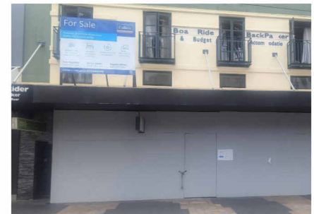
Reference Photo - Existing awning
