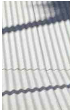
MR - METAL ROOF CUSTOM ORB PROFILE. COLOUR TO MATCH EXISTING. COATING SUITABLE FOR SEA-SIDE ENVIRONMENT.
