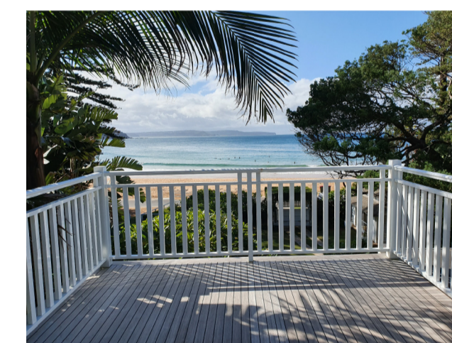
7. Alum. balustrade and window frames Powder coat finish To match existing Manufacturer - Dulux Colour - White Satin
