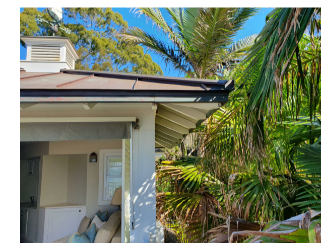
6. Ribbed Copper roof To match existing
