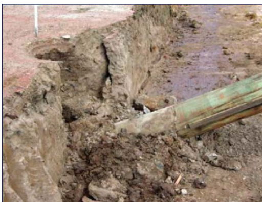
Excavation causing pole collapse
