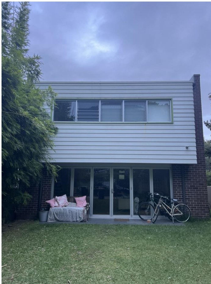
Figure 5. The rear of existing dwelling, looking west from the rear yard/parking
