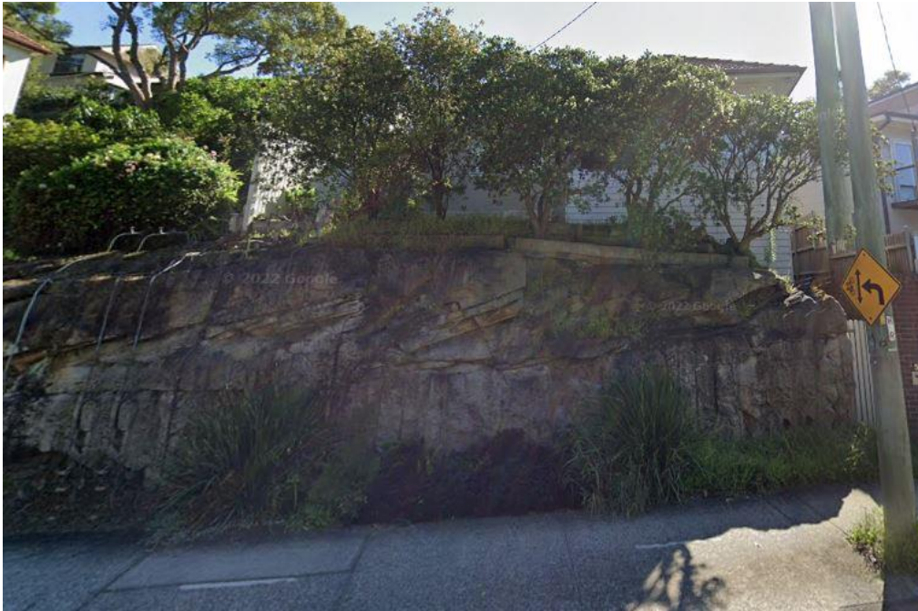
Figure 4. The front of existing dwelling, looking east, view from Pittwater Road.
