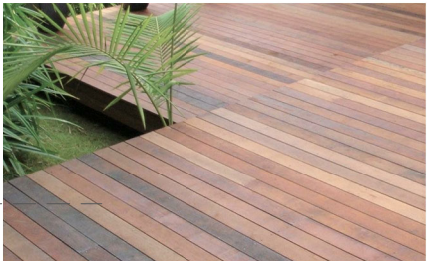
timber deck - spotted gum decking - natural finish
