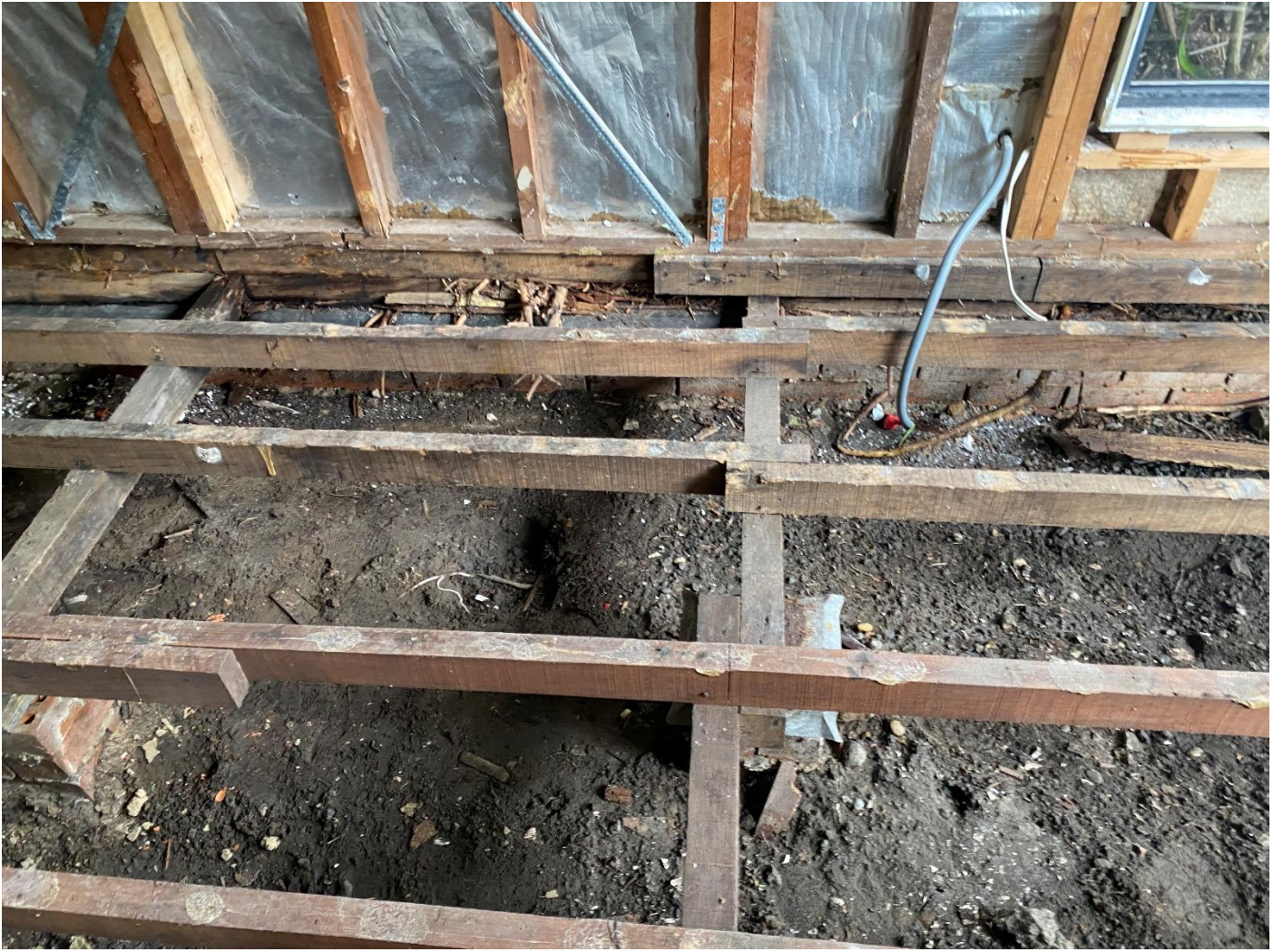
Internal Timber Framing of South West Wall and Floor
