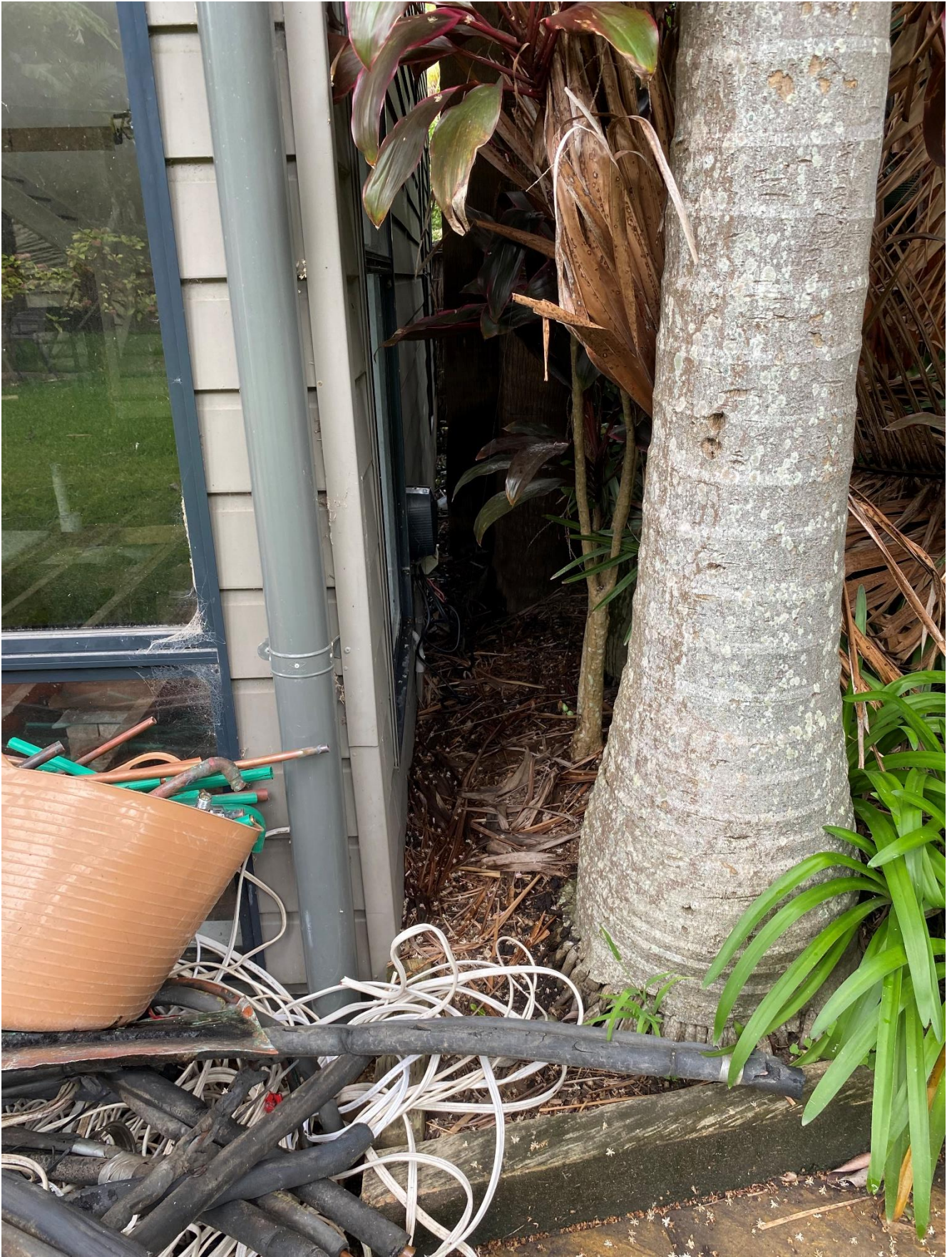
External view of South west Wall
