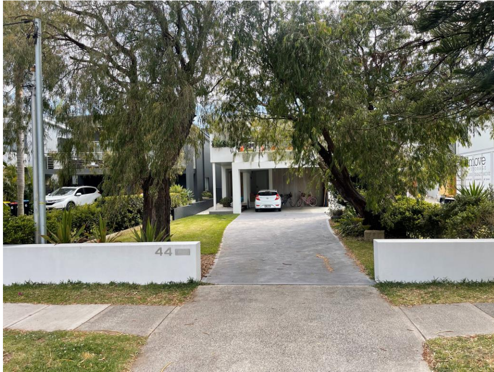
Fig 2: View of the subject site from Kooloora Avenue, looking north-east
