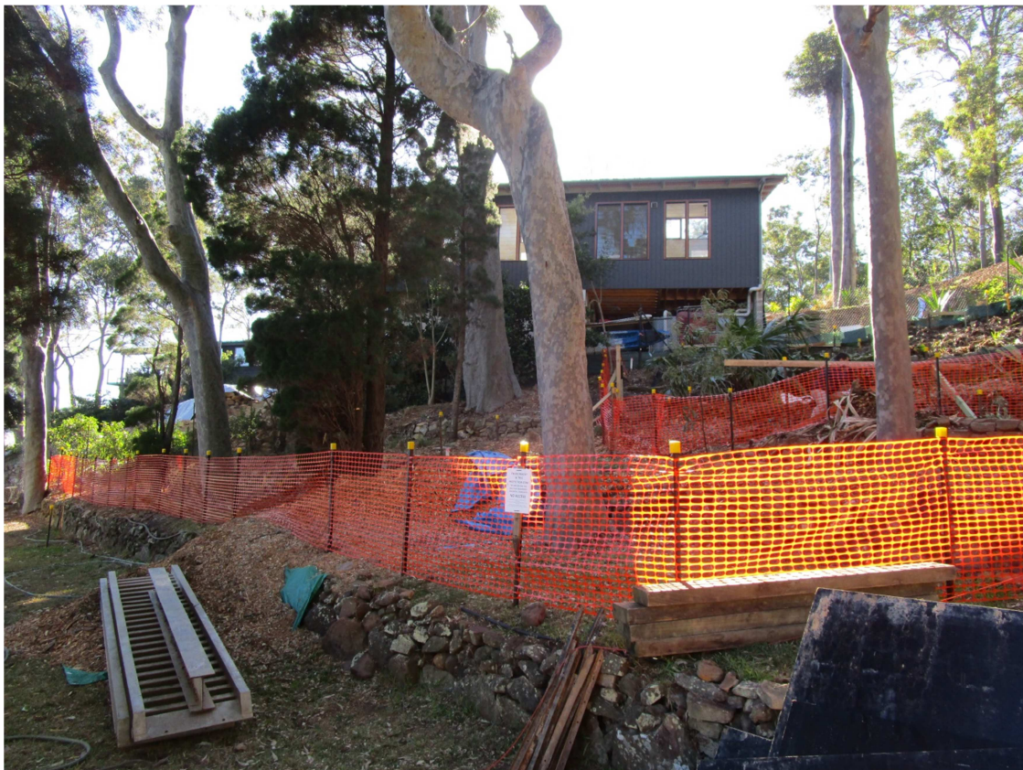
Figure 2: Site photo taken on 1 st of August 2018, showing the Tree Protection Zone fencing around the subject Tree
