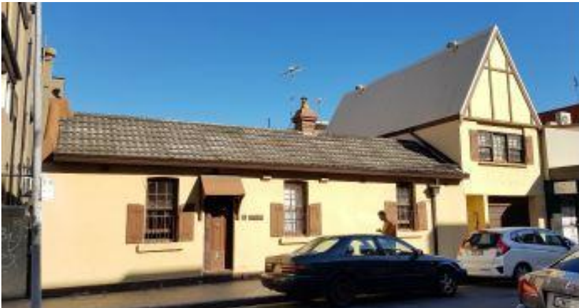
EXISTING COTTAGE ON SITE 21 WHISTLER STREET
