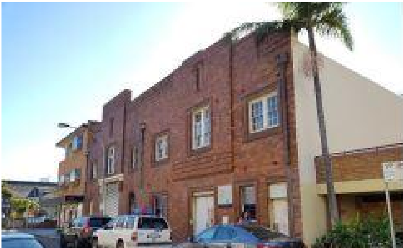
No.33 MANLY SUBSTATION
