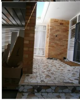
Similarly, the new Laundry and Toilet shows only the works that are infill of the old windows....the floor, ceiling and roof in this area are all to be retained. New walls are to be built over the existing walls as existing windows are removed to allow for the new Laundry and Toilet layout.
