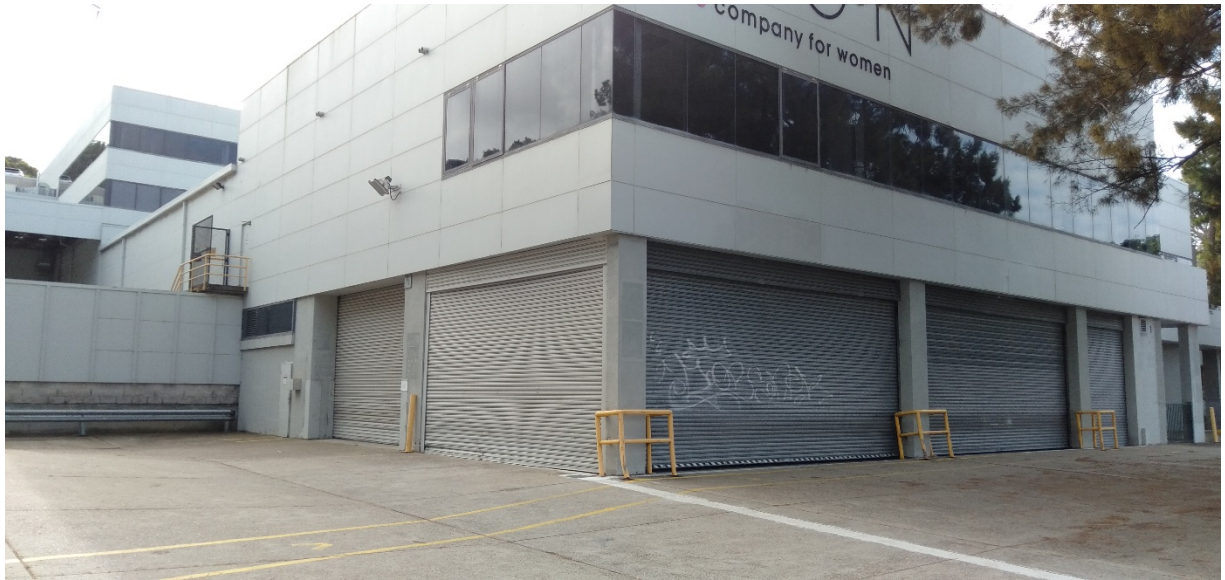
Photo 1: 2-Storey Distribution Centre at Southeast corner of the site
