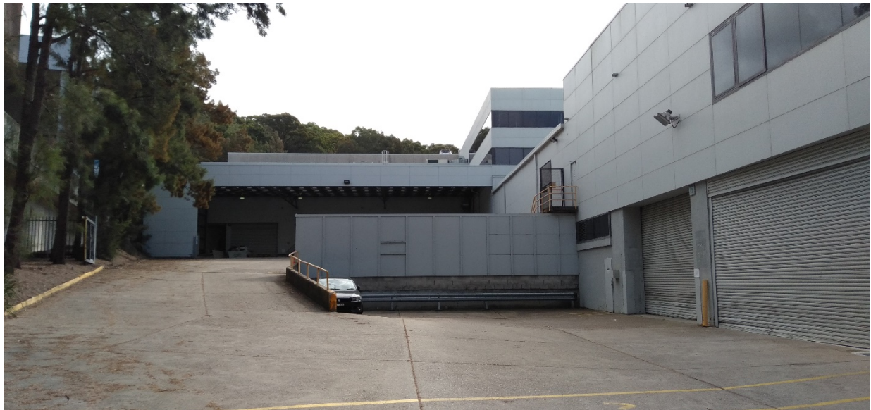
Photo 2: Ramp up to level 1 loading dock of 5-storey Office and Warehouse building at Southeast corner of the site
