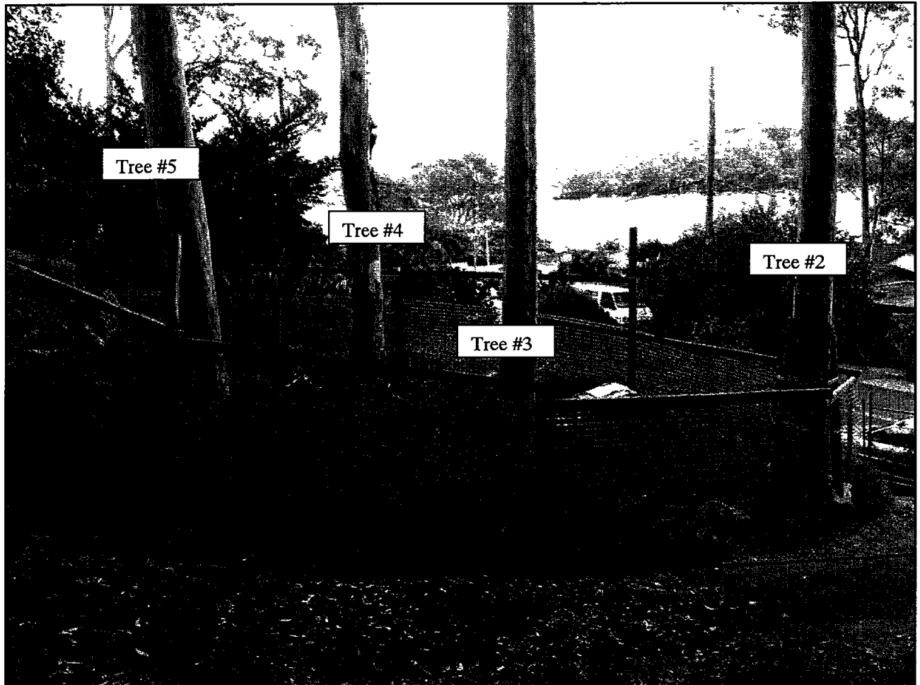
Figure 1: Illustrates TPZ installation, note “Tree Guard” installed around trunk of Tree #2
