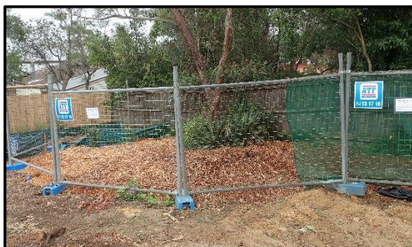
Image 1: Good tree protection fencing as per AS 4970 – 2009. Image Paxton
