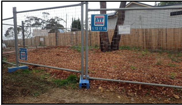
Image 3: Good tree protection fencing as per AS 4970 – 2009. Image Paxton.
