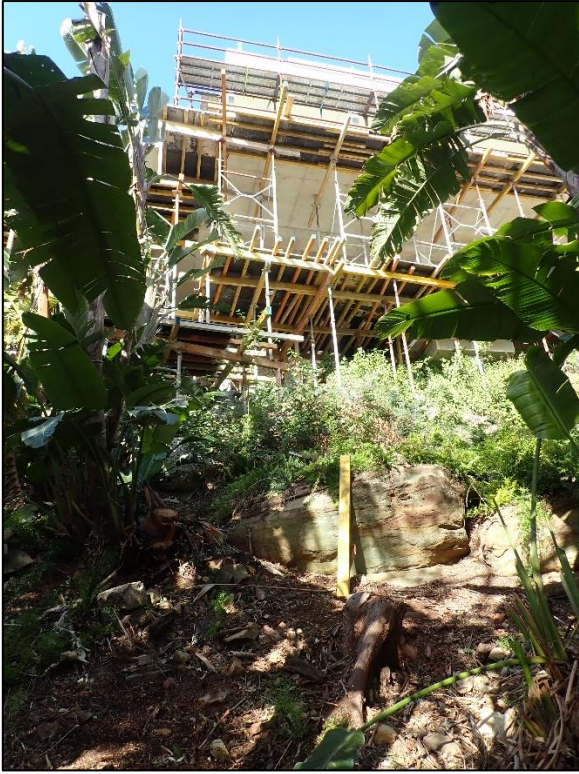
Image 6, Approximate location of inclinometer.
