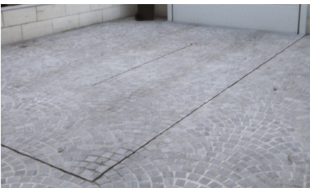
Synthetic stone covering (3 cm thick)
