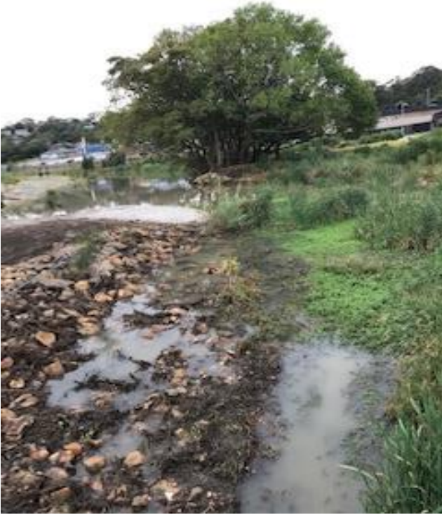
Upstream obstruction causing creek to back up
