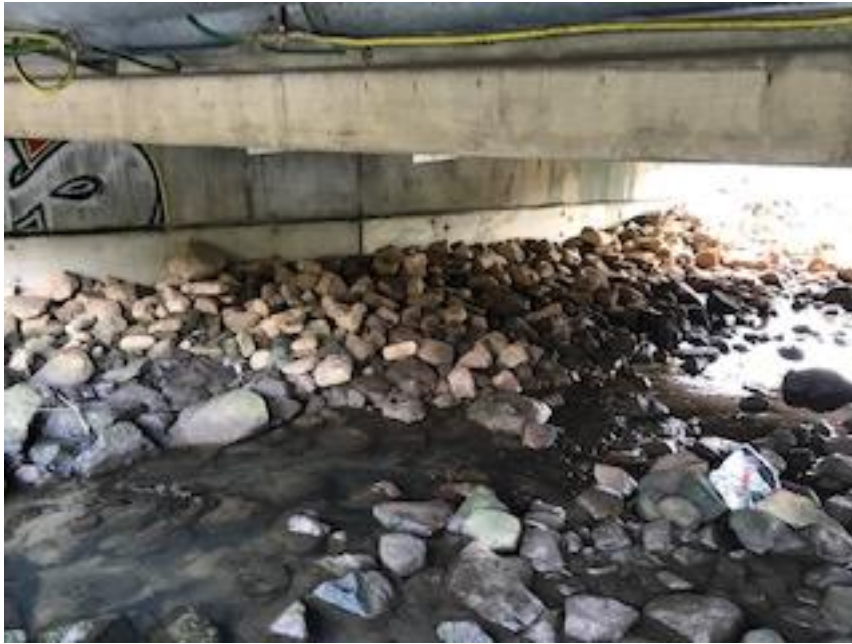
Obstruction in the culvert
