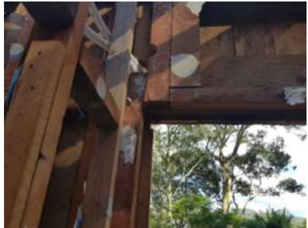
Photo 2: Inadequate stud framing adjacent window opening.
