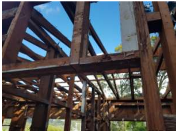
Photo 2: Inadequate stud framing adjacent window opening.
