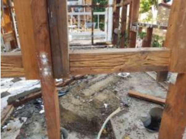
Photo 7: Example of termite damage to framing.
