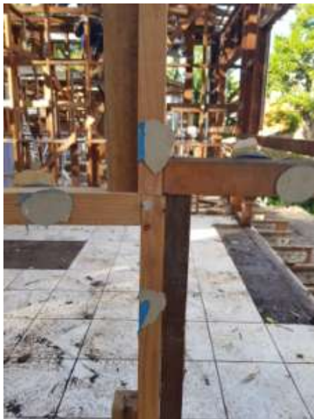
Photo 3: Example of stud cut in two separate pieces
