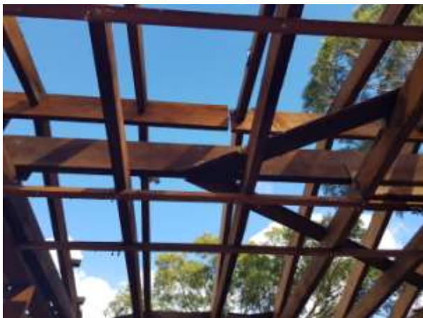
Photo 5: Discontinuous roof ridge member.
