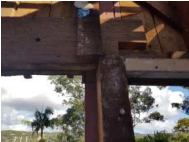
Photo 1: Inadequate stud framing adjacent window opening.
