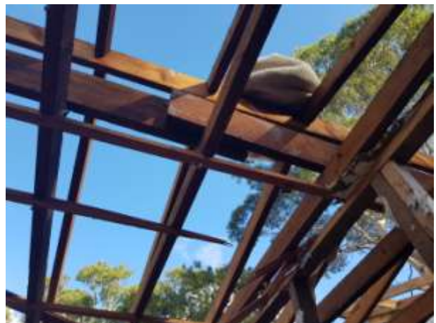
Photo 6: Ceiling hanging beams not adequately supported.
