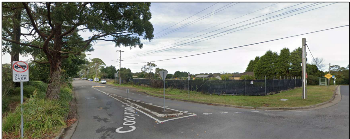
Figure 6: Subject site viewed from corner of Cooyong and Myoora Roads looking south-east towards the site (source: Google Maps)
