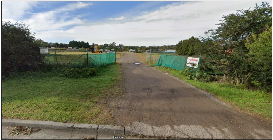
Figure 12: Looking east from Myoora Road looking towards adjoining southern property at 279 Mona Vale Road (source: Google Maps).
