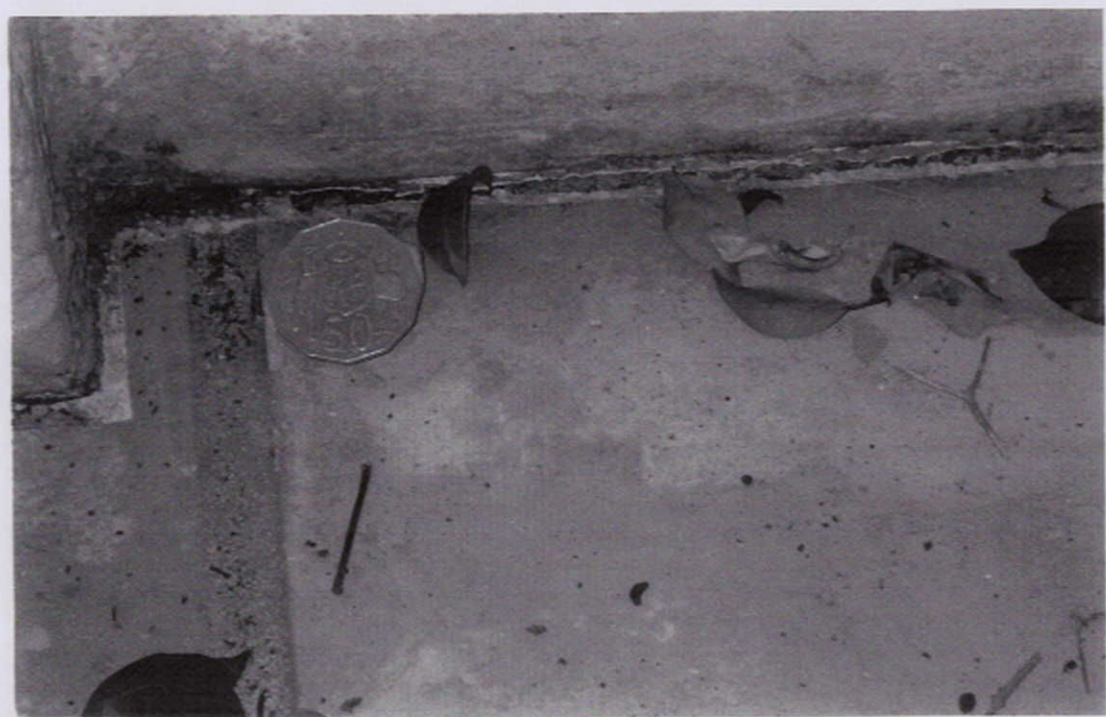
Settlement Cracking at Base of Eastern Boundary Wall Viewed East
