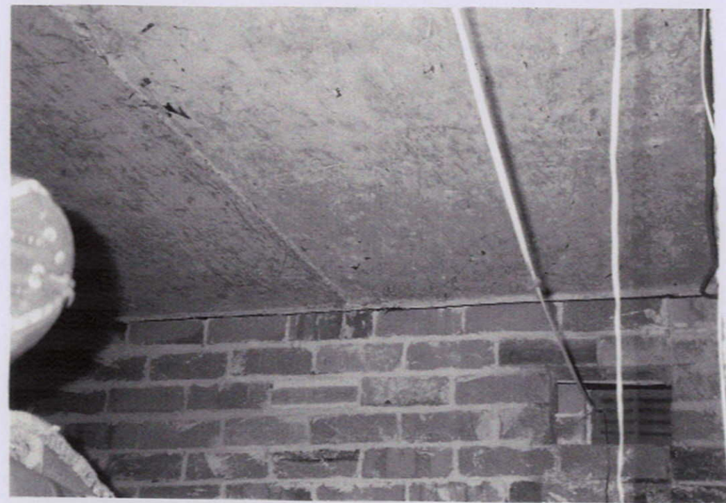
Western Brickwork Viewed West SubFloor Garage Level. No Expansion Cracking due to the Render to Brickwork.
