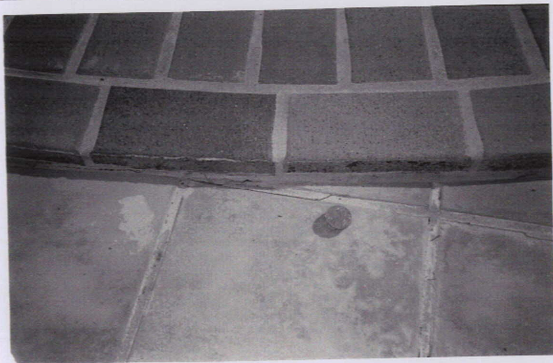
Settlement Cracking around pool edge to Copping / Tile intersection
