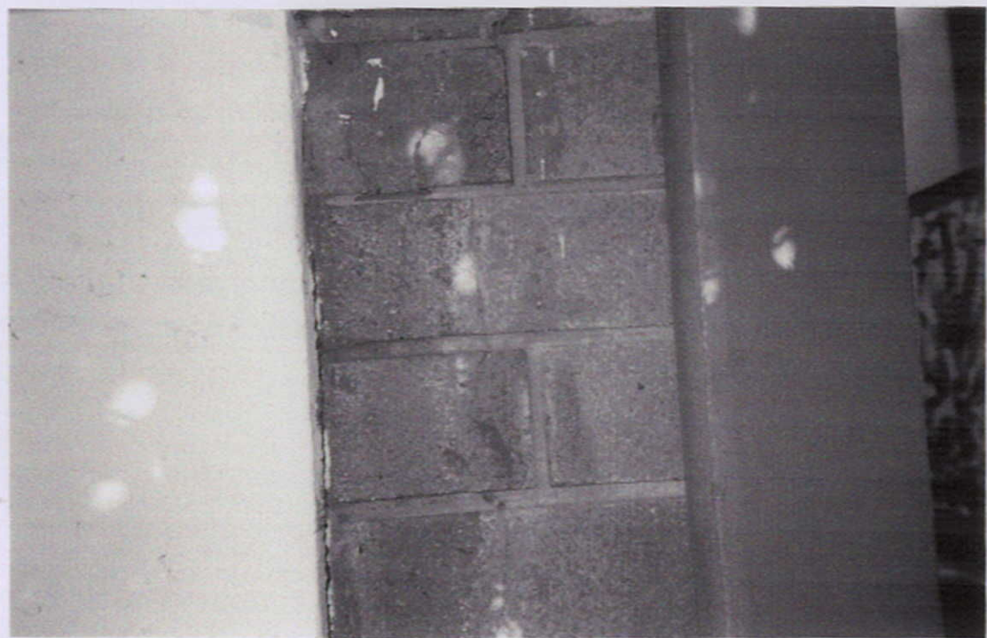
Minor Cracking to Pier Front of House at Garage Level Viewed South East Boundary End.
