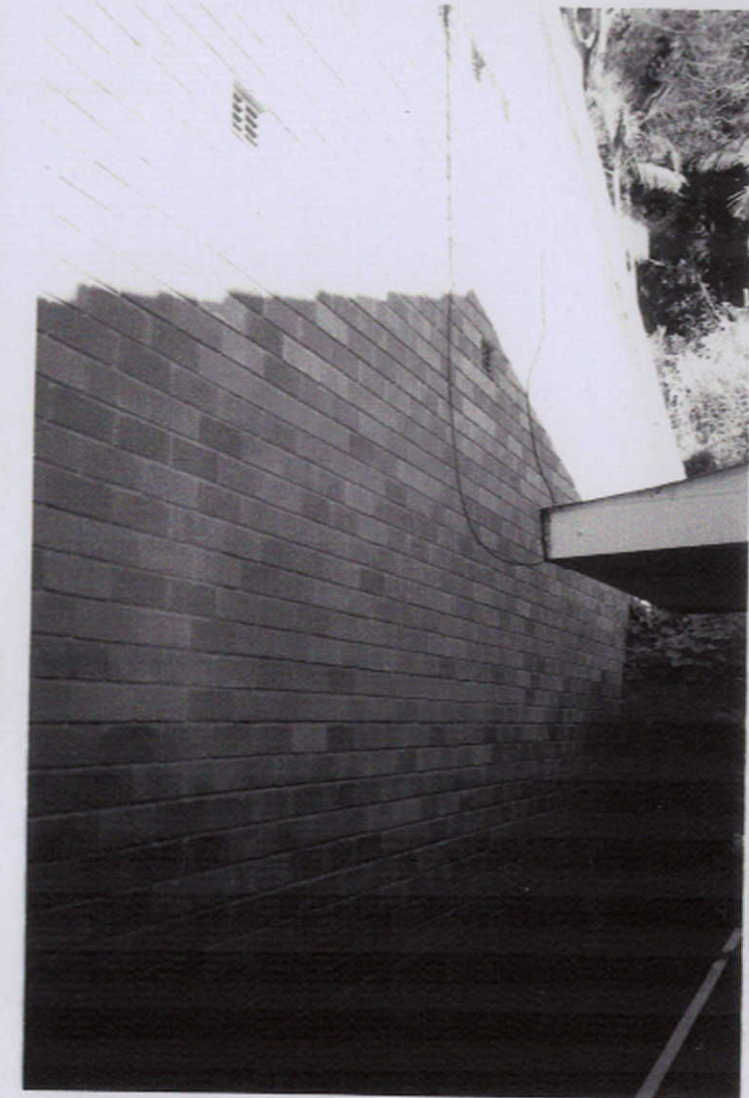
② Western Brickwall Viewed South East
