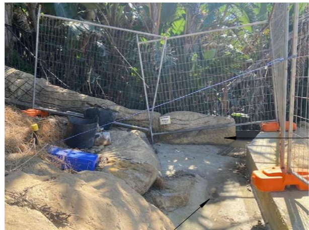
concrete drain across back of piers and capping beam
