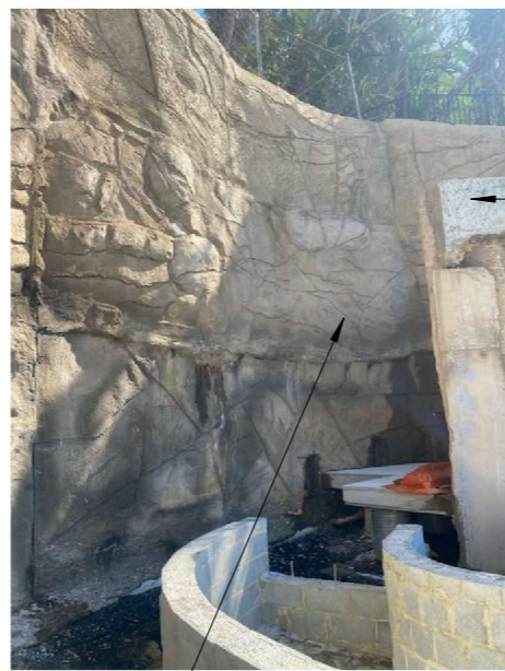
rise for inclinator to replace stairs
