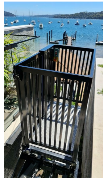
inclinator car detail
