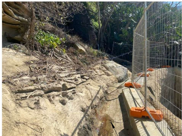
concrete drain across back of piers and capping beam
