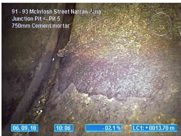
, 00:04:47, 13.60 Displaced joint, radial displacement, radial displacement: 11-20mm at 5 o'clock
