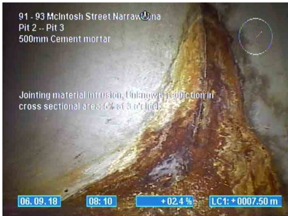
, 00:03:16, 7.50 Jointing material intrusion, Unknown, reduction in cross sectional area: 5% at 3 o'clock
