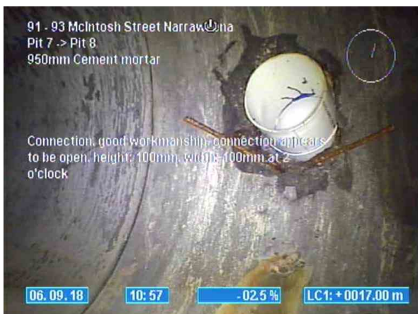
, 00:03:03, 17.00 Connection, good workmanship, connection appears to be open, height: 100mm, width: 100mm at 2 o'clock
