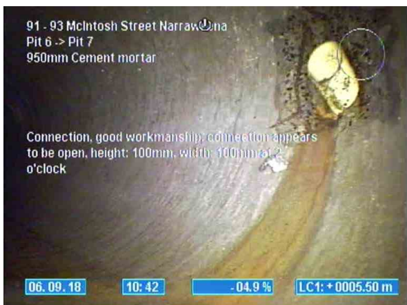
, 00:05:04, 5.50 Connection, good workmanship, connection appears to be open, height: 100mm, width: 100mm at 2 o'clock
