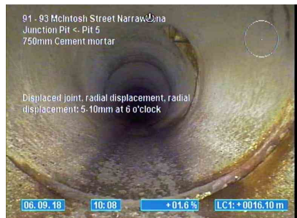
, 00:06:23, 16.10 Displaced joint, radial displacement, radial displacement: 5-10mm at 6 o'clock
