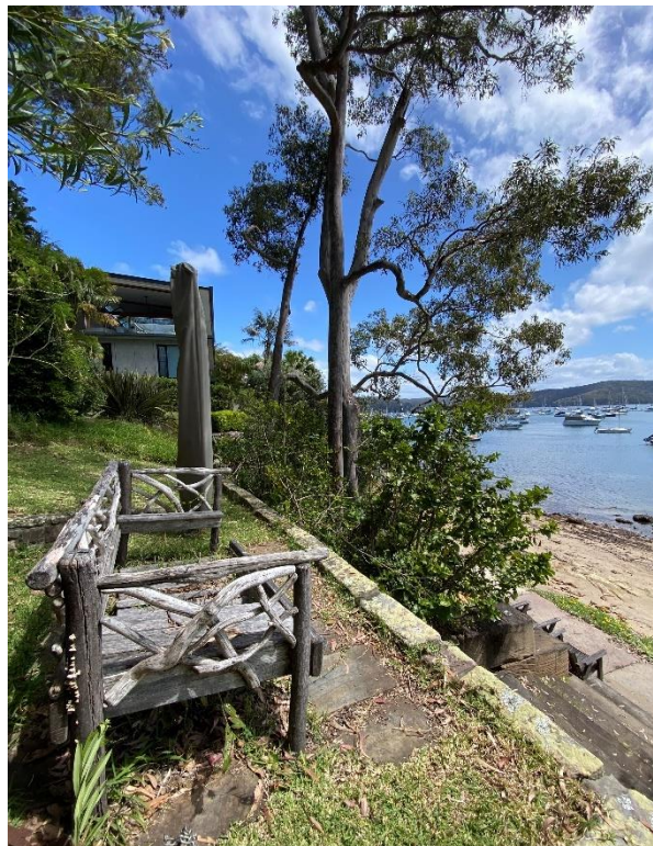
Photo 4: View of existing retaining walls, looking south-west
