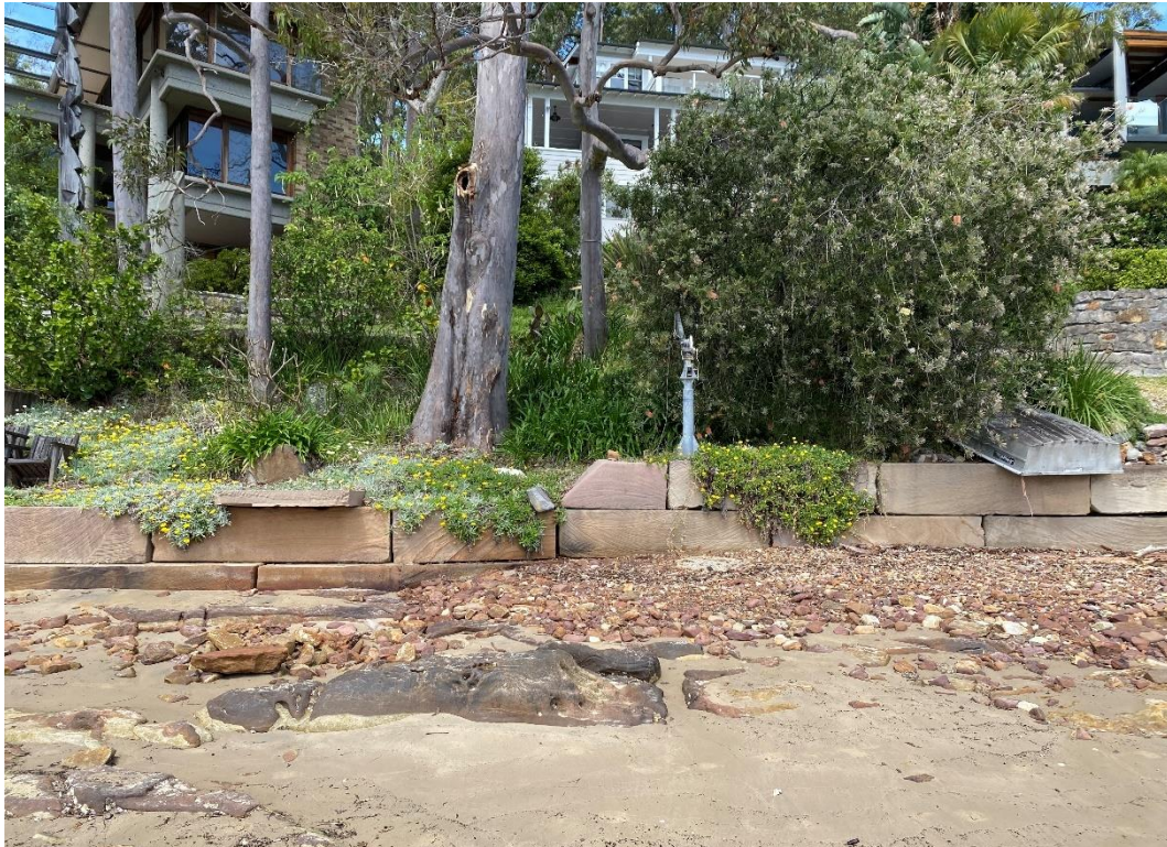
Photo 3: View of the site from the Pittwater foreshore, looking south-east
