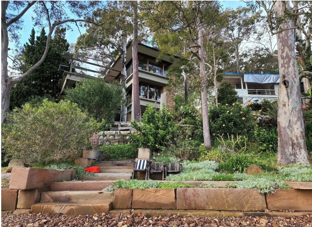
Photo 5: View of the site from the Pittwater foreshore, looking east
