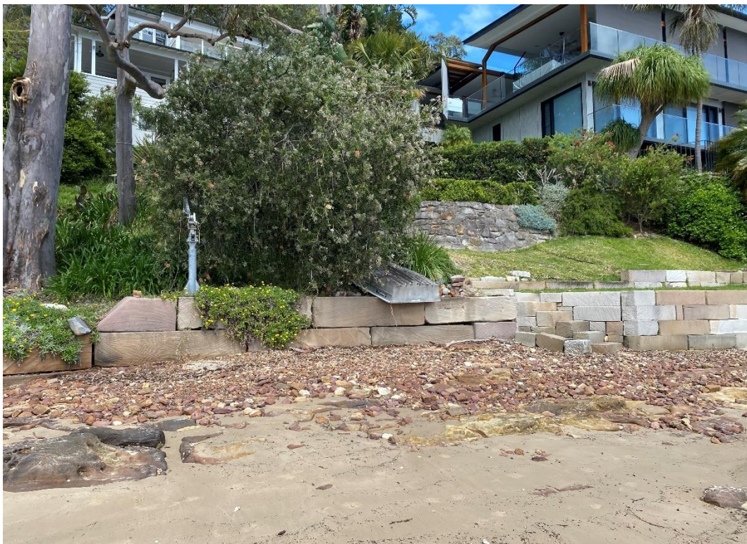
Photo 2: View of the site from the Pittwater foreshore, looking south-east
