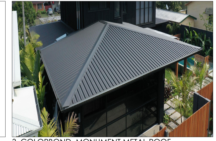
3. COLORBOND MONUMENT METAL ROOF
