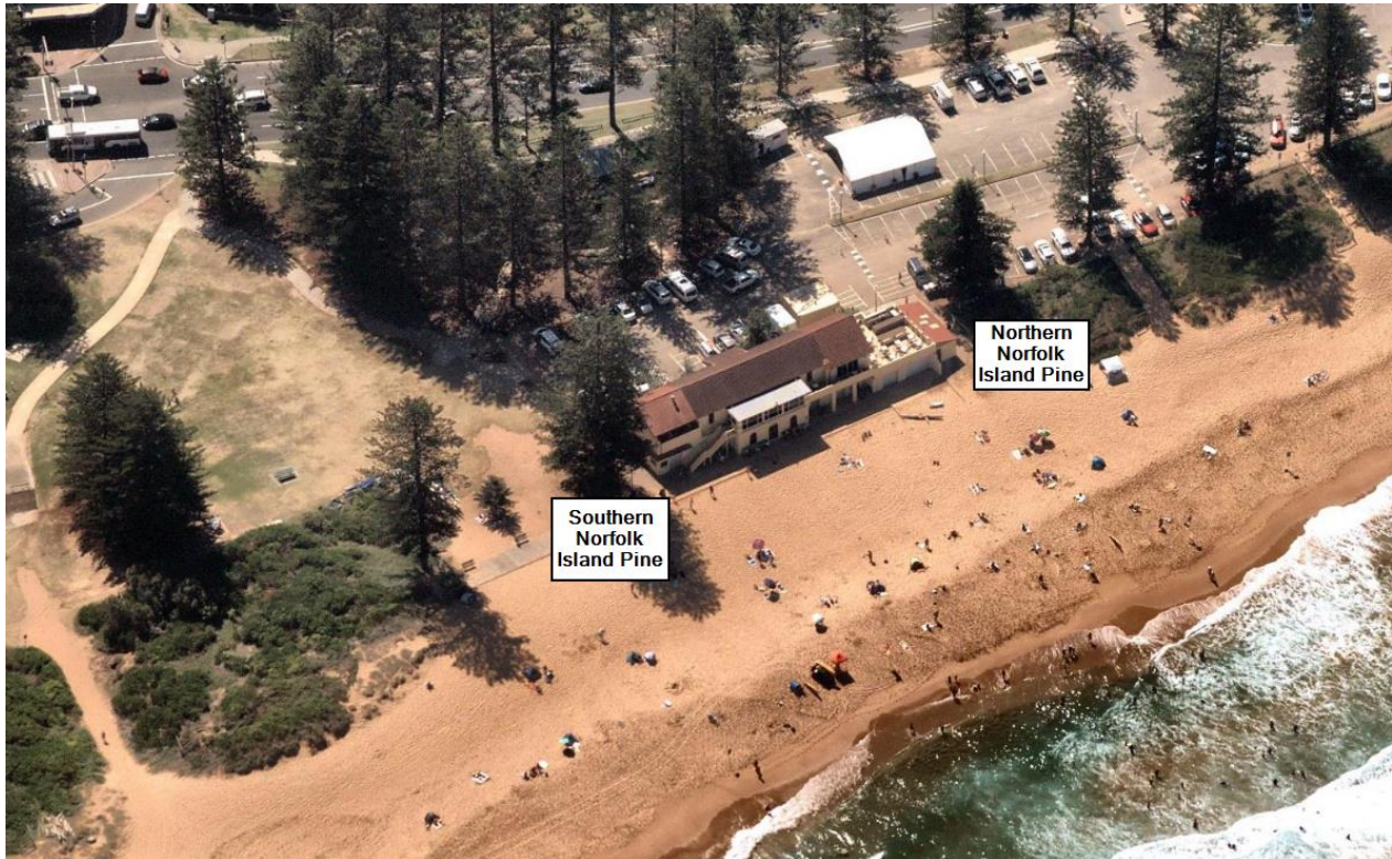
Figure 2-2 Oblique aerial view of Newport SLSC showing the two significant Norfolk Island Pine trees (source: HCE, 2021a)
