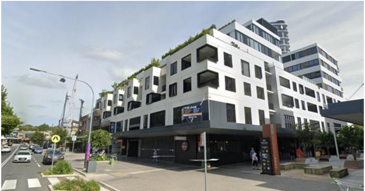
Figure 3: Meriton Lighthouse development located on the northern side of Oaks Avenue opposite the subject site with 4 storey podium
