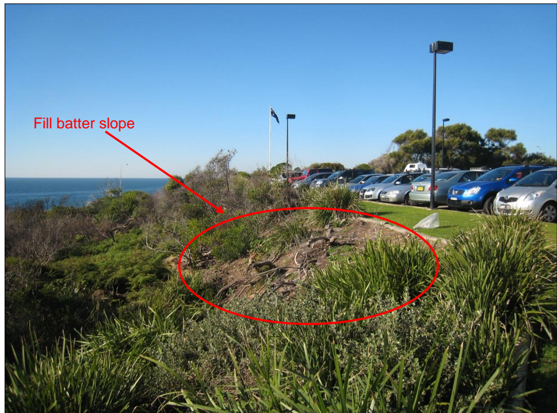
Plate 2: Fill batter slope along northern side of AC car park
