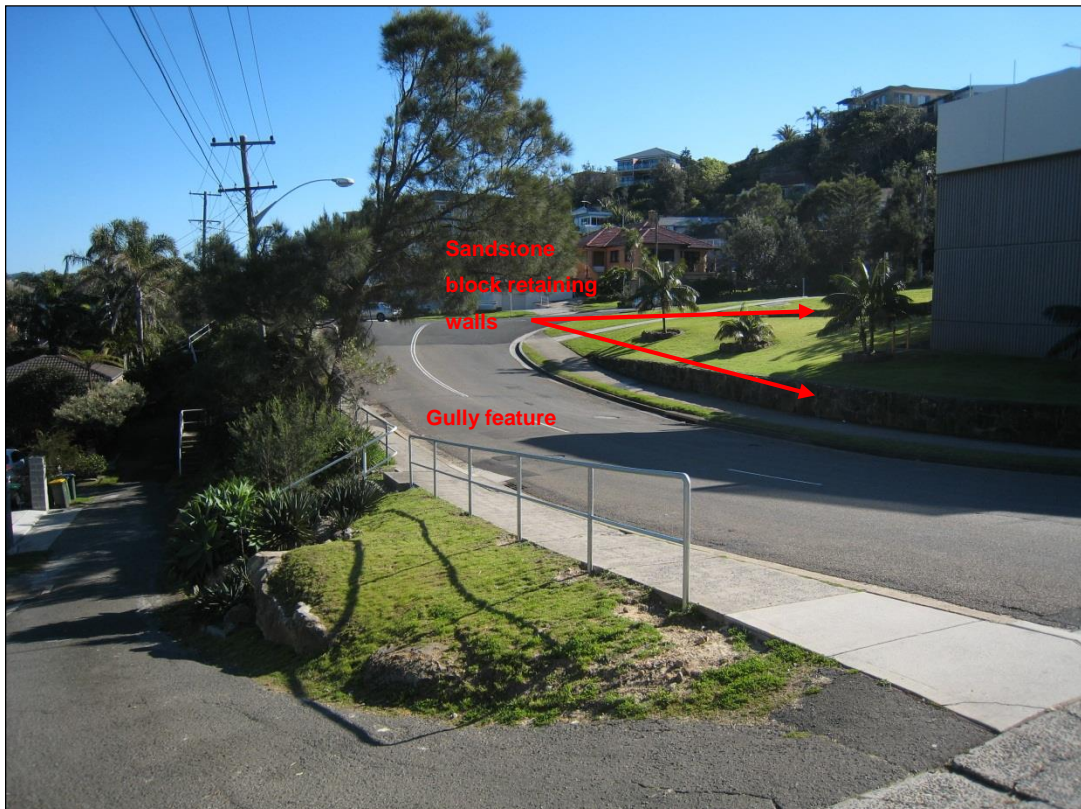
Plate 6: View looking across Evans Street towards the south-western corner of the site, showing low height mortared sandstone block retaining walls and a shallow gully feature.
