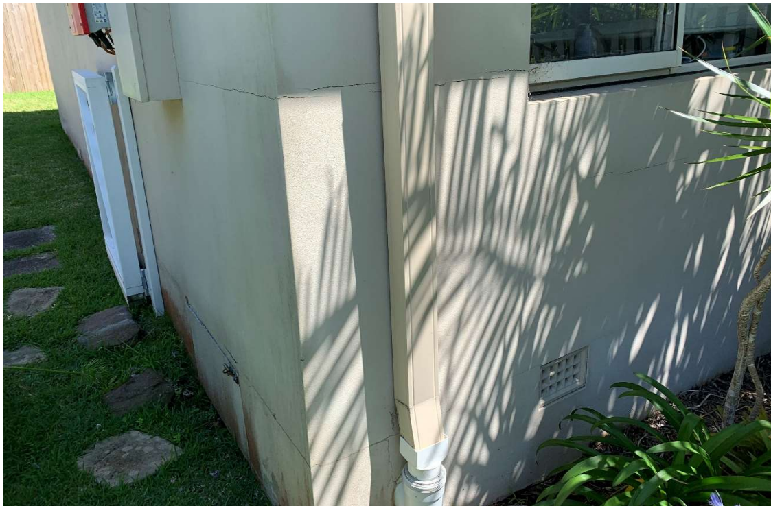
Photograph 5: Horizontal cracking within south eastern corner of structure, facing north west
