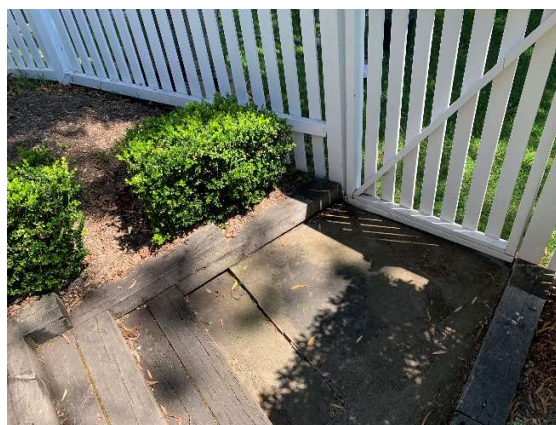
Photograph 4: Movement within the pavers due to underlying roots of the adjacent gum tree, facing north west
