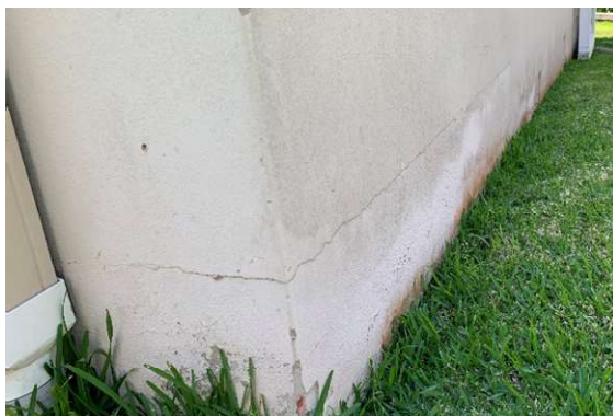
Photograph 6: Cracking within south western corner of structure, facing north east
