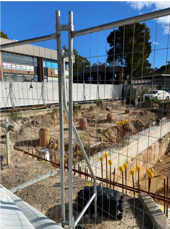
Figure 9 – Looking south east towards subject site. Adjacent site currently under construction.
