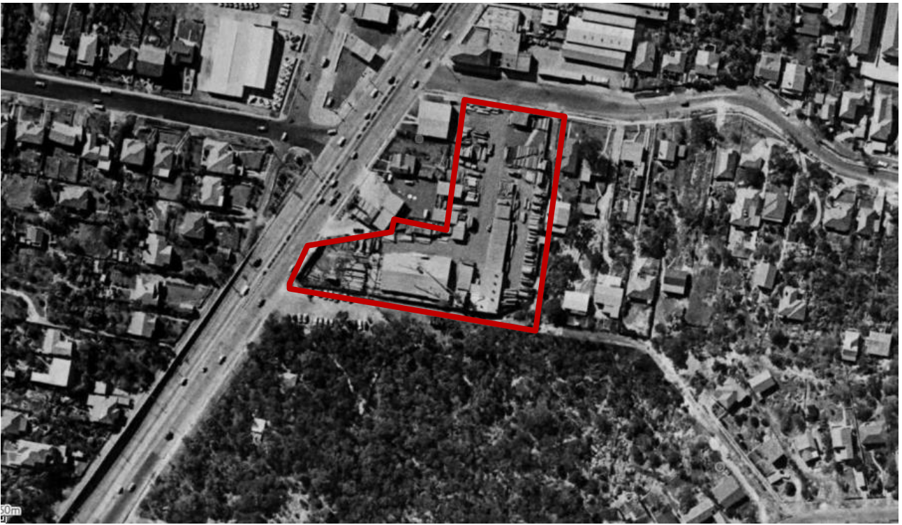
Figure 22 – 1965 Aerial showing approximate location of subject site outlined in red. Note: Earlier industrial sheds appear constructed on the subject site.
