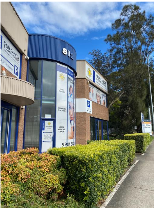
Figure 15- Front façade of subject site located at 812 Pittwater Road.
