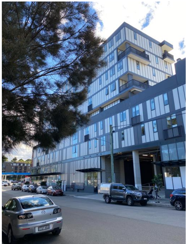
Figure 6 – Looking north west towards building located on opposite side of Delmar Parade.
