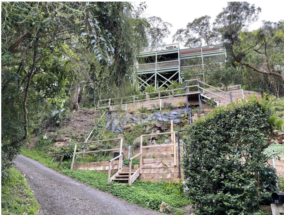
Figure 5: Stairs to the front of the dwelling and front of the existing dwelling
