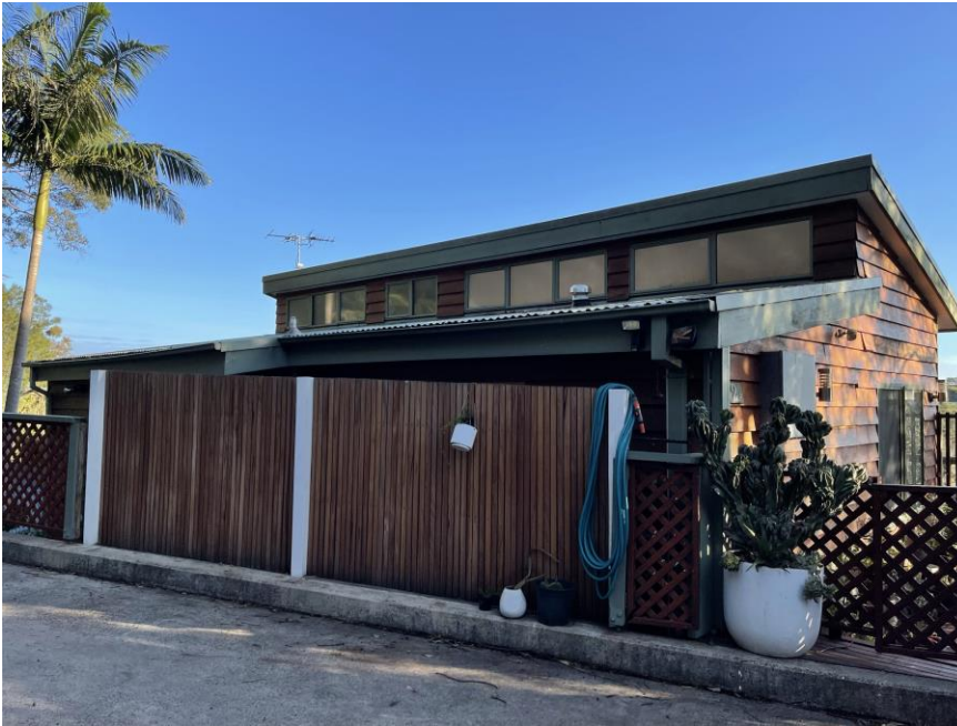
Figure 8: Rear of the existing dwelling
