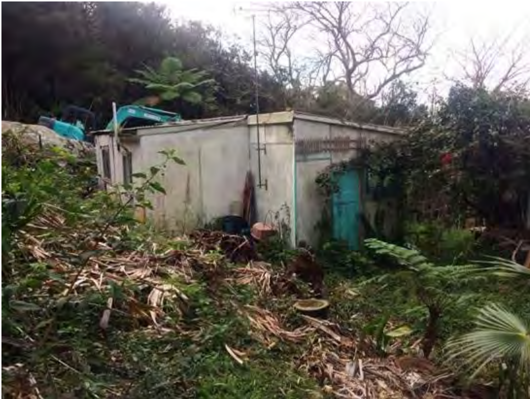
Photograph 4.10 Old shed on the Subject Site
